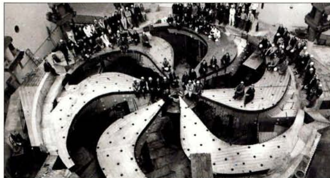
The TRIUMF cyclotron magnet, half-complete, in January 1972.
